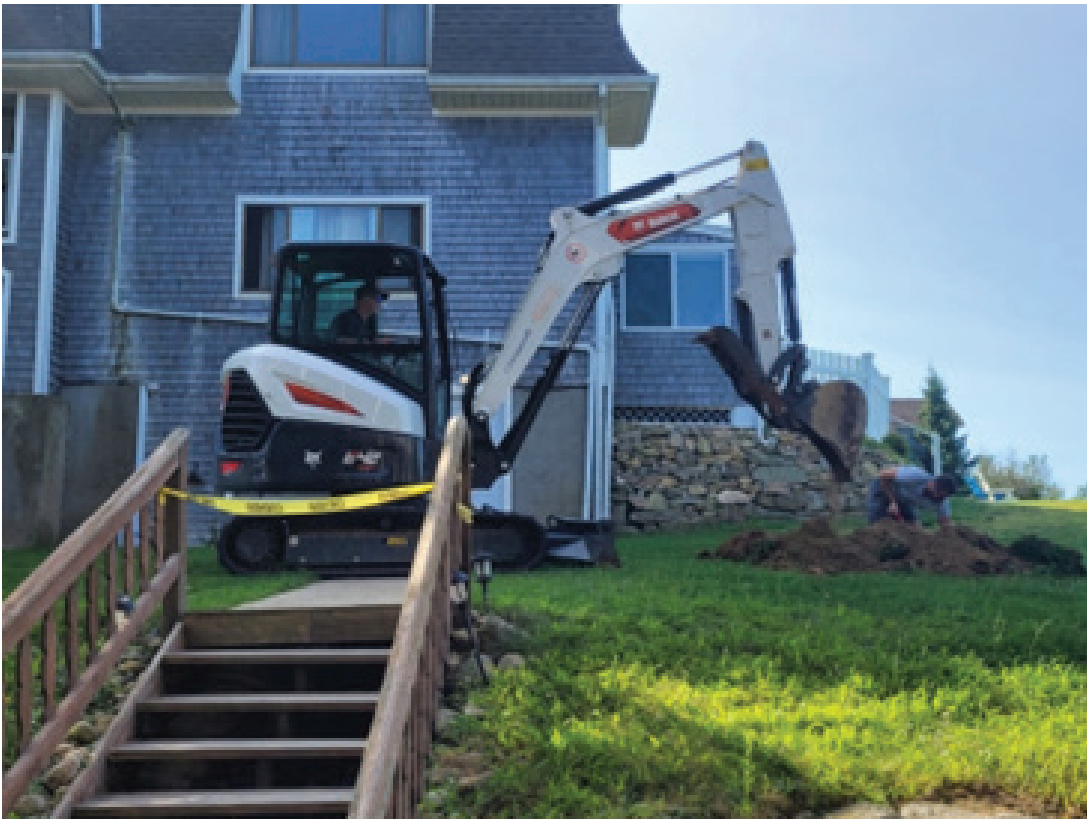
Digging the Trench for Bldg. A Sewer Line Replacement
