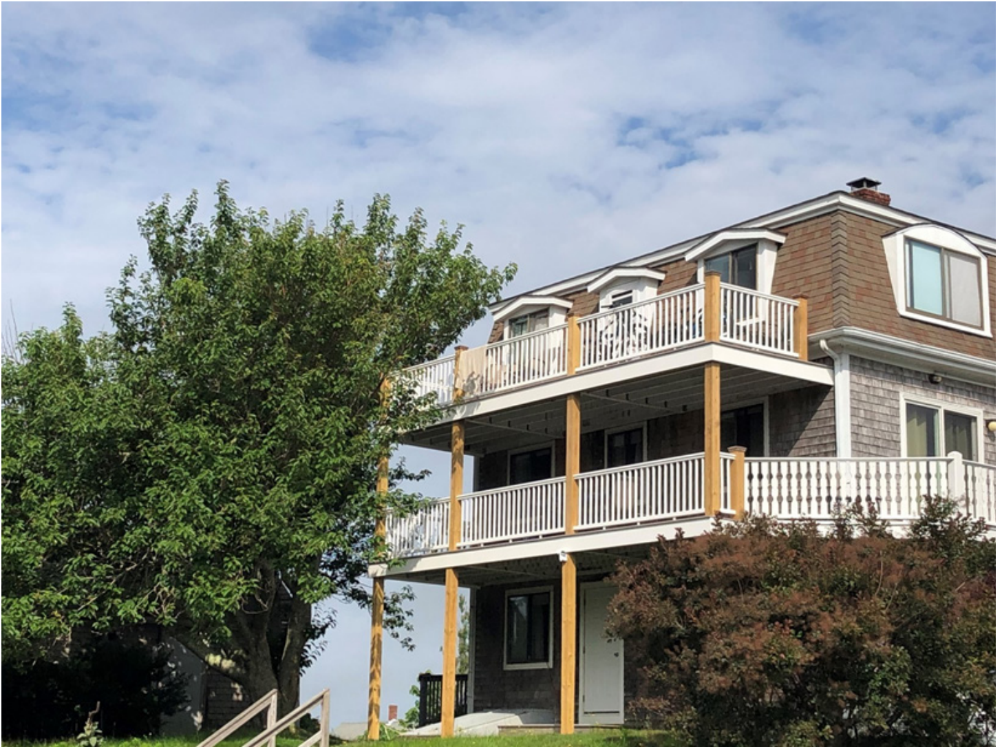
The New Decks of Units 7 and 14
