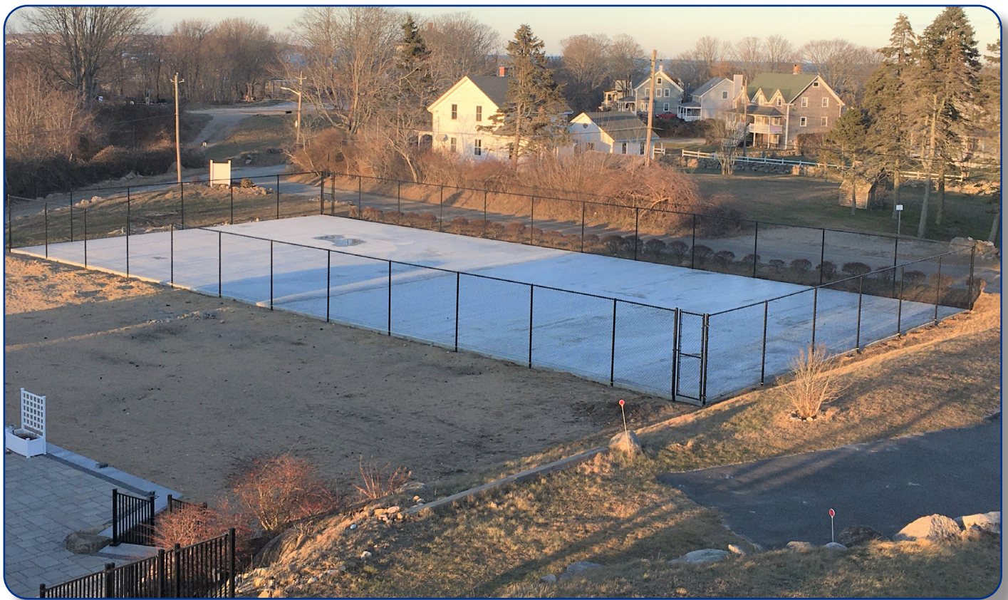
New Tennis Court Under Construction
