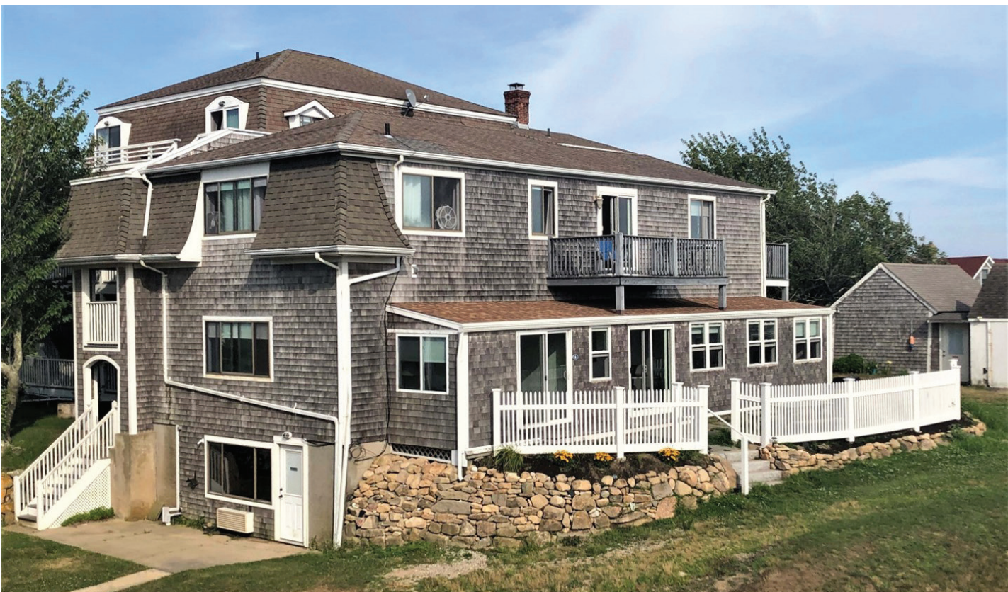
New Fence, Stairs, and Retaining Wall Immediately Behind Units 4, 5, and 6
