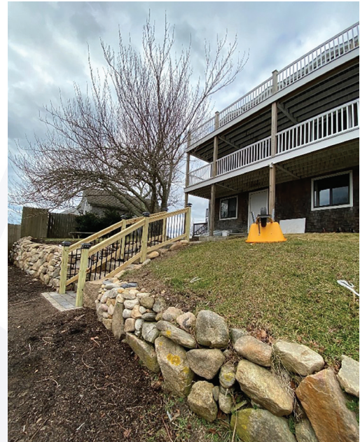
New Wall & Stairs between Bldg. A and Shed
